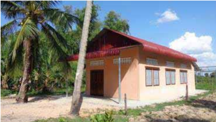
The school is Solar powered with a water well and 2 toilets
