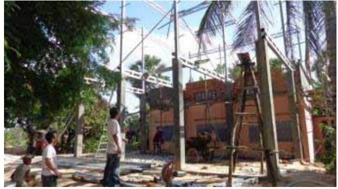
Steel frame workers now erecting the upper storey
